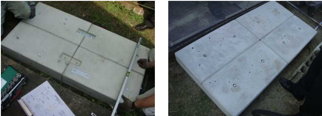
Fig 3: Pre-cast base for Ene-Farm
